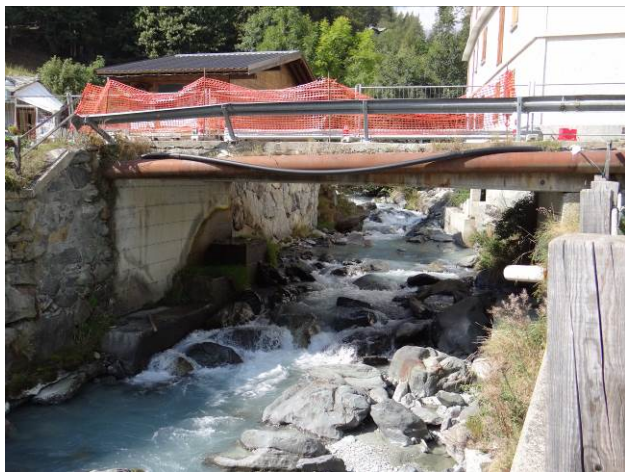
Ponte strada Balme-Fraz. Cornetti
