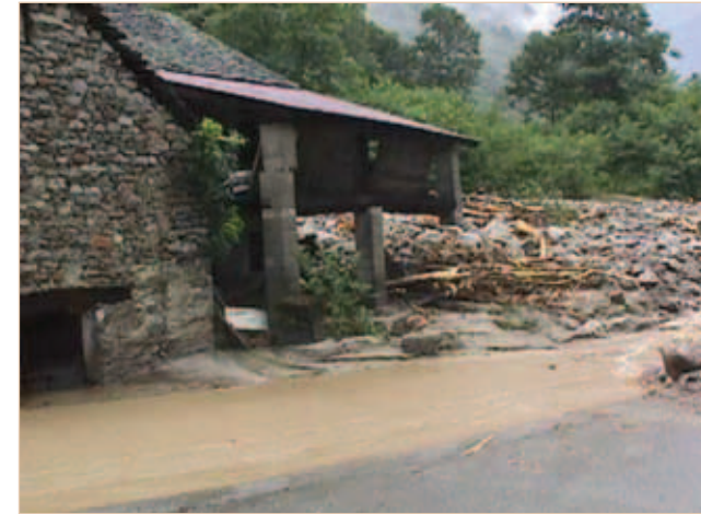
Figure 4.2.2.C/1.3 A house on the road surrounded and flooded by water and debris, Cassinello Torrent, 4 July 2000.
