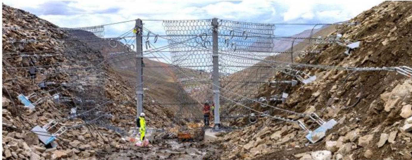
Figure 7 shows installation of 7 m high posts at net 13 on 19 th of August 2024. The horizontal ropes and retaining ropes are connected to the Flexheads/anchors but the work on the ring net is still under way. The photo also shows how fractured and loose the Svalbard rock and soil is. Photo: Arni Jonsson.
